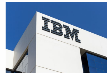
IBM Data Center , Spain
